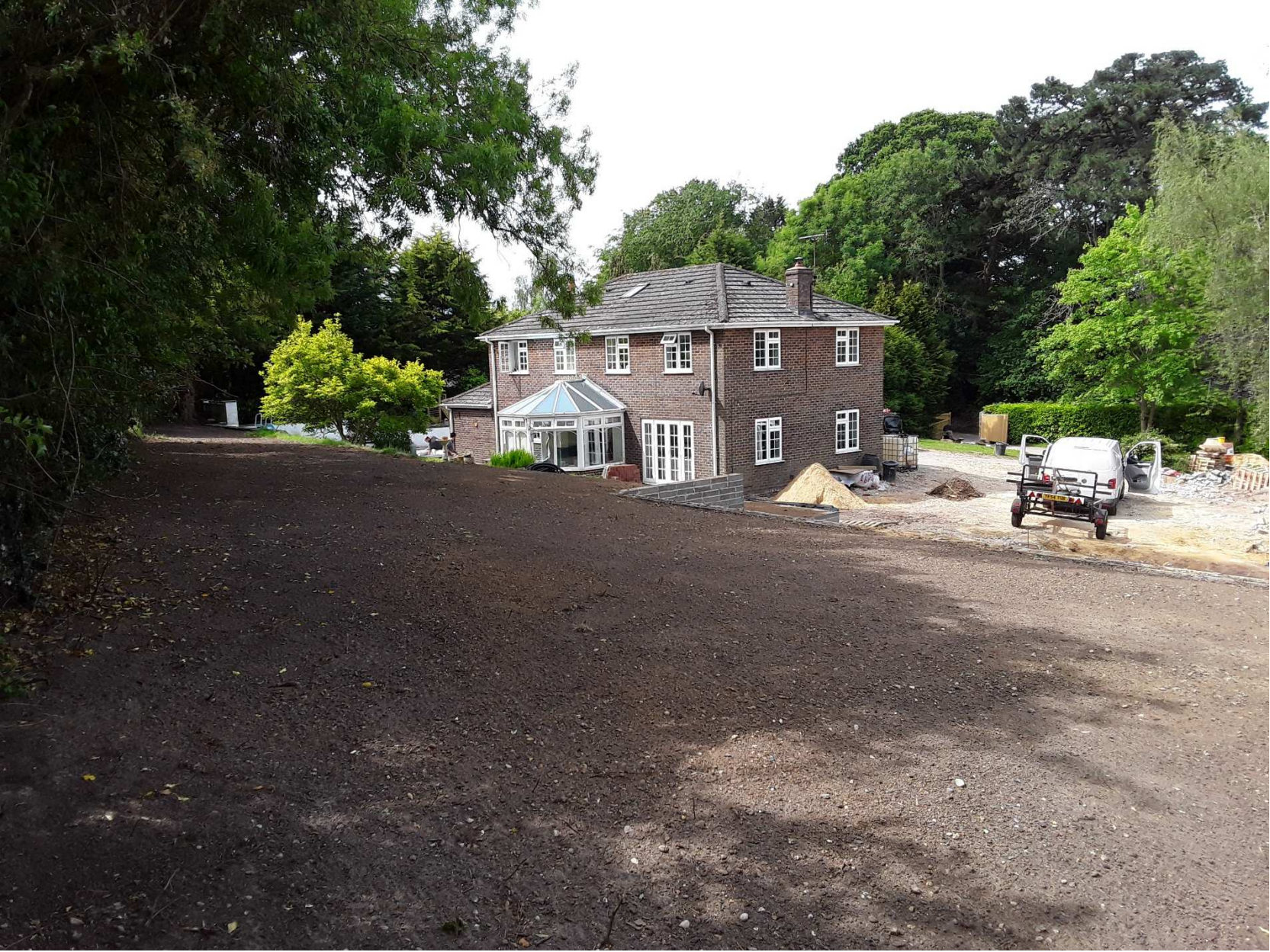
View back towards rear of existing property
